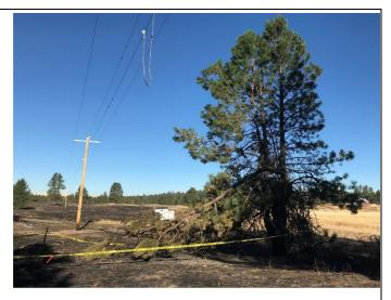
The power pole to the west of this section of power lines was resting on the ground partially suspended by the power lines and the lower portion of the wood pole was missing. I noticed the mild predominate wind was out of the northeast at the time of our arrival, which is consistent with the previous day's expected high winds.
